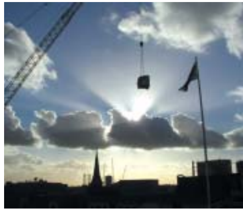
The magnet of the Siemens MAGNETOM Symphony scanner is being hoisted into the Middlesex Hospital by crane.
